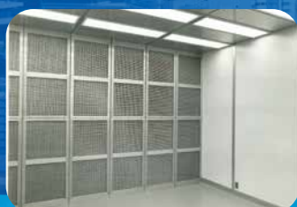
Takasago laminar flow cleanroom
