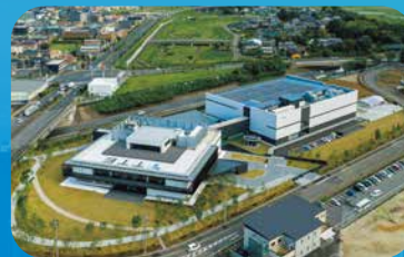
Takasago Thermal Engineering Innovation Center
