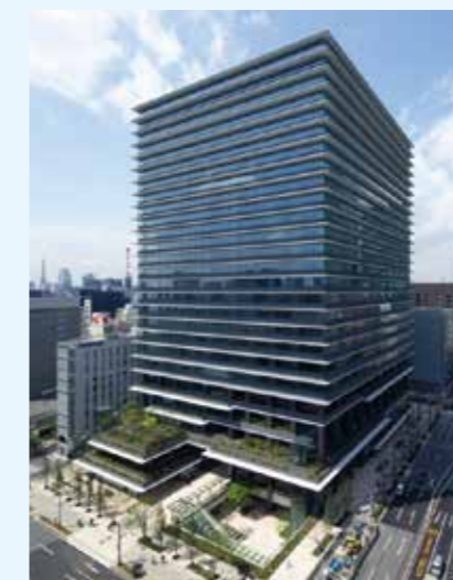
Tokyo Square Garden (Society of Heating, Air-Conditioning and Sanitary Engineers of Japan Award: 54th Technical Award, Building Equipment Category)
