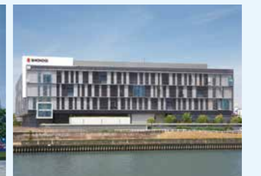
Shionogi Pharmaceutical Research Center (Society of Heating, Air-Conditioning and Sanitary Engineers of Japan Award: 52nd Technical Award, Building Equipment Category)
