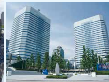
Makuhari Techno-Garden (Society of Heating, Air-Conditioning and Sanitary Engineers of Japan Award: 3rd Special Award, Renewal (Renovation) Award)
