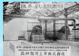
1927 Rayon plant temperature and humidity conditioning equipment (Teijin Iwakuni) Building Mechanical and Electrical Engineering Heritage No. 15
