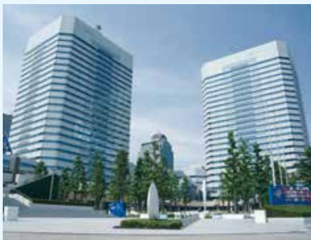
Makuhari Techno-Garden (Society of Heating, Air-Conditioning and Sanitary Engineers of Japan Award: 3rd Special Award, Renewal (Renovation) Award)
