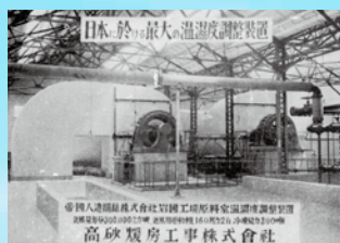
1927 Rayon plant temperature and humidity conditioning equipment (Teijin Iwakuni)
