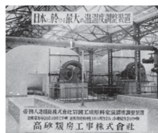
1927 Japan's first Precised temperature and humidity Control System (Iwakuni Plant of Teikoku Rayon Co., Ltd. (current Teijin Limited))
