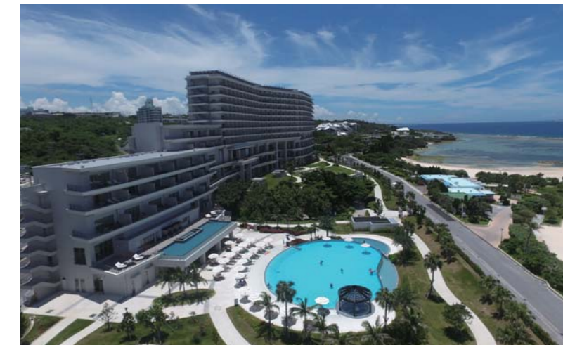
Hotel Orion Motobu Resort & Spa:Received the 32nd Promotion Award (Technology Promotion Award) given by the Society of Heating, Air-Conditioning and Sanitary Engineers of Japan and the 6th Carbon Neutral Award
