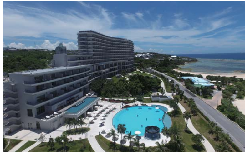
Hotel Orion Motobu Resort & Spa:Received the 32nd Promotion Award (Technology Promotion Award) given by the Society of Heating, Air-Conditioning and Sanitary Engineers of Japan and the 6th Carbon Neutral Award
