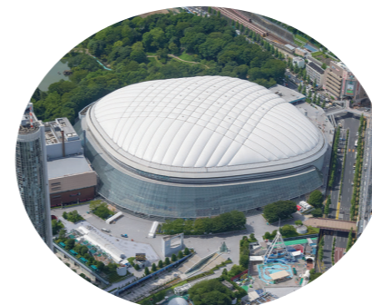
1988 Tokyo Dome Air conditioning of Japan's first air-supported dome stadium Photo courtesy of Tokyo Dome Corporation
