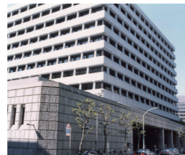
1973 The New Building of the Bank of Japan's Head Office Source: Bank of Japan
