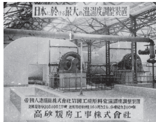
1927 Japan's first Precised temperature and humidity Control System (Iwakuni Plant of Teikoku Rayon Co., Ltd. (current Teijin Limited))
