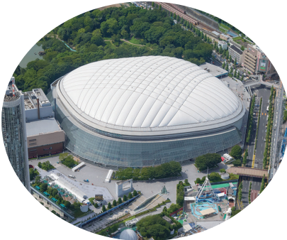
1988 Tokyo Dome Air conditioning of Japan's first air-supported dome stadium Photo courtesy of Tokyo Dome Corporation
