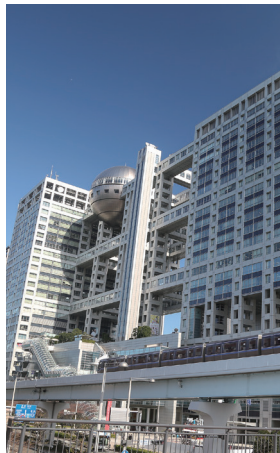
1996 Head office building of Fuji Television Network, inc. 2005 Developed a swirling induction type HVAC system, SWIT®
