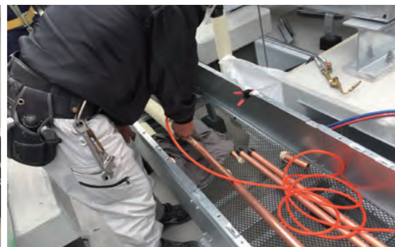
Construction work to apply the EI-brazing method
