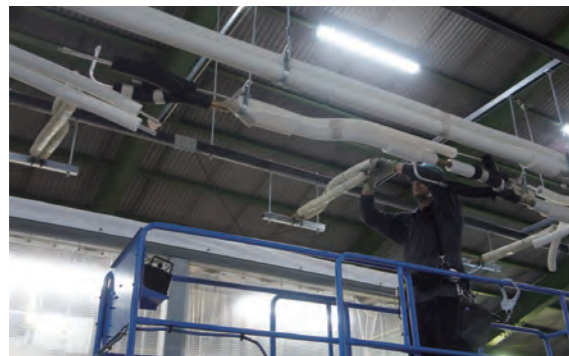
Installation of aluminum refrigerant pipes
