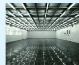
1968 Cleanroom that was also able to be used for semiconductor production (TCR Super MP)
