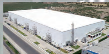
Project name: TDS Battery Factory & Warehouse Project Use: On-vehicle lithium-ion battery plant Client's name: TDS Lithium-Ion Battery Gujarat Private Limited Purchaser's name: SMCC Construction India Limited Area /Country: Gujarat, India
