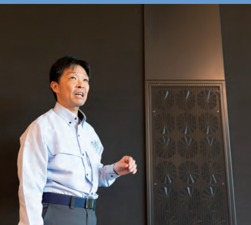
Displacement air conditioning panel SWIT® installed on the walls of the cafeteria
