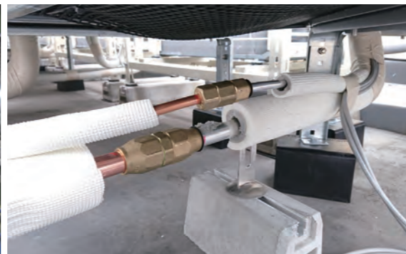
Installation of mechanical joints for aluminum refrigerant piping
