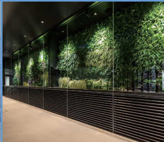
Outdoor air inlets installed on the exterior wall
