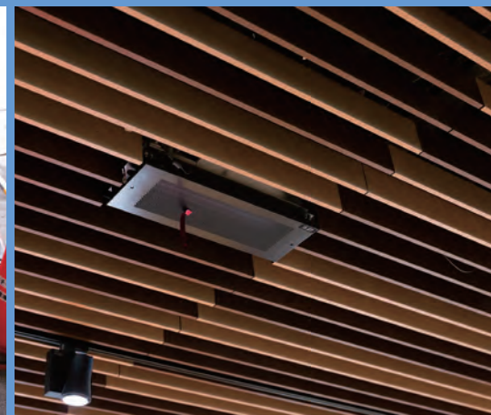
Air conditioner for individual use (DCFCU) that allows users to control the setting according to their preference
