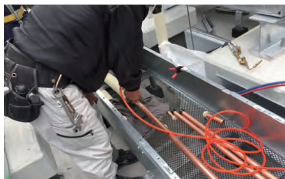
Construction work to apply the EI-brazing method
