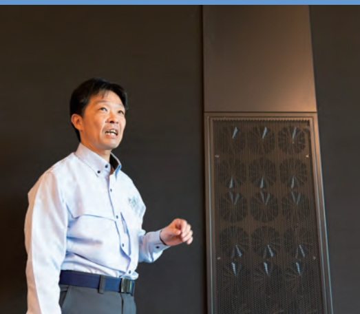
Displacement air conditioning panel SWIT® installed on the walls of the cafeteria
