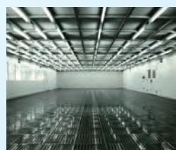
1968 Cleanroom that was also able to be used for semiconductor production (TCR Super MP)
