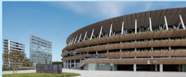
2019 National Stadium Photo courtesy of Taisei Corporation
