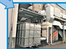
In-plant industrial air conditioning (painting process) → Reduction in dehumidification and heating load
