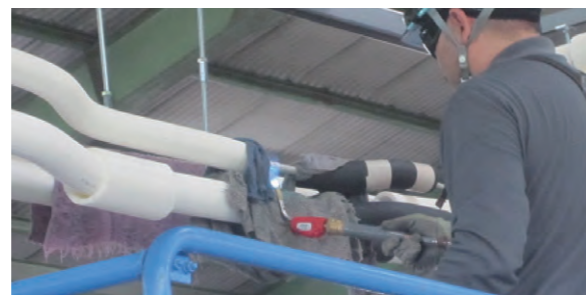
Aluminum pipes brazing work
