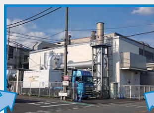
In-plant cogeneration system → Recovering heat from exhaust gas (160°C) and exhaust warm water (80°C)
