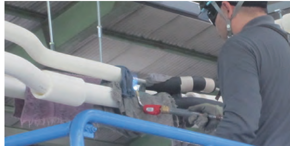
Aluminum pipes brazing work
