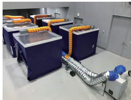
Full view of the anti-COVID-19 air-conditioning and ventilating booth for anti-disaster shelters
