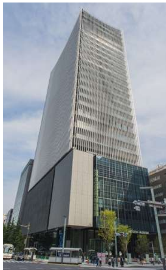
Realization and demonstration of an open-plan skyscraper for Museum Tower Kyobashi Received the 36th Award for Promotion of Technology from the Society of Heating, Air-Conditioning and Sanitary Engineers of Japan
