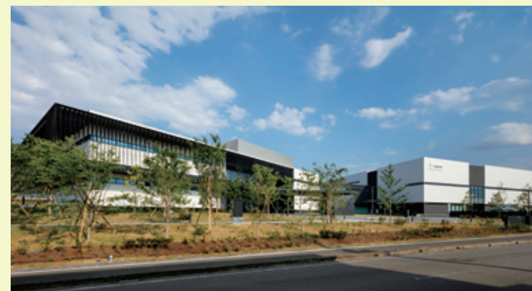
■ Panoramic view of the building
