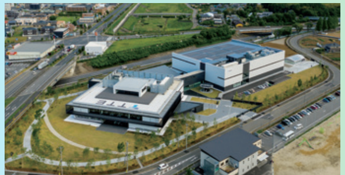
Takasago Thermal Engineering Innovation Center
