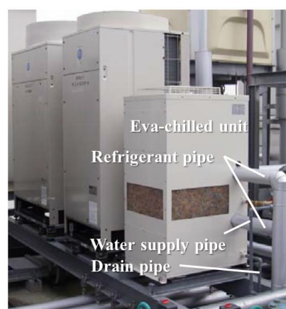
Fig. 1 Eva-chilled unit when installed in the PAC's outdoor unit.
