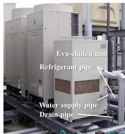
Fig. 1 Eva-chilled unit when installed in the PAC's outdoor unit.
