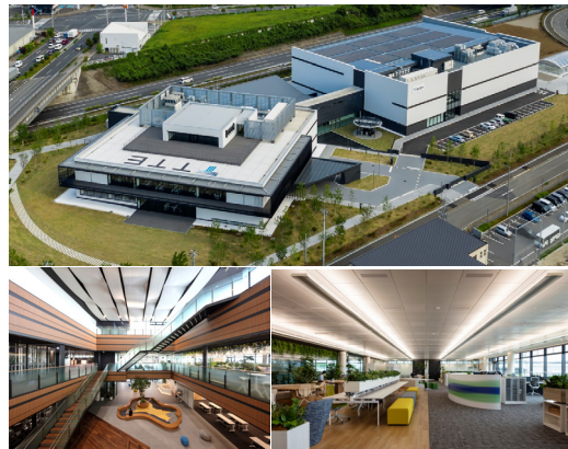
Fig. 1 Exterior (upper) & interior (down) view of the facility
